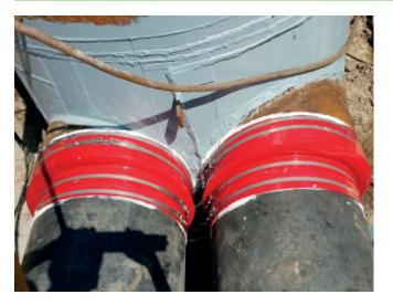
**Pipe movements and settings** are the big challanges for a **pipeline wall penetration seal**, especially at **pre-isolated warm-going pipelines**.
