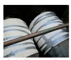
Before backfilling protect sealing sleeves with expansion-pads
